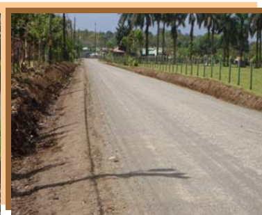
Cruce San Jorge-El Tanque
